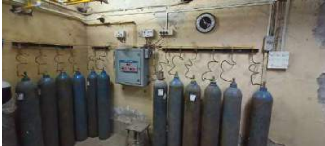
SITC of Manifold, Header Bars, Tail Pipes: Liquid Oxygen (Cryogenic Dura Cylinders) Stainless Steel Manifold Supply System of 10+10 size : 10cylinder manifold bank as left side and 10cylinder manifold bank as right side
